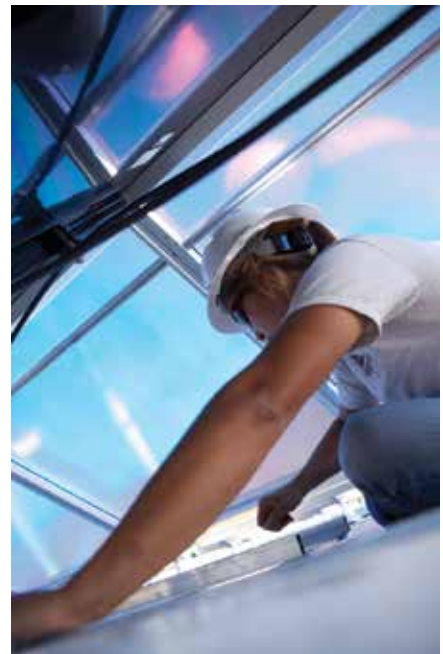
LEFT: Designed to bring power to those in need, a solar trailer belonging to the Shonto Community Development Corporation has mounted panels on the roof and a battery and control console inside. ROGER CLARK ABOVE: An 80KW solar photovoltaic system being installed at Leupp High School, Leupp, Arizona. DANIEL SNYDER
