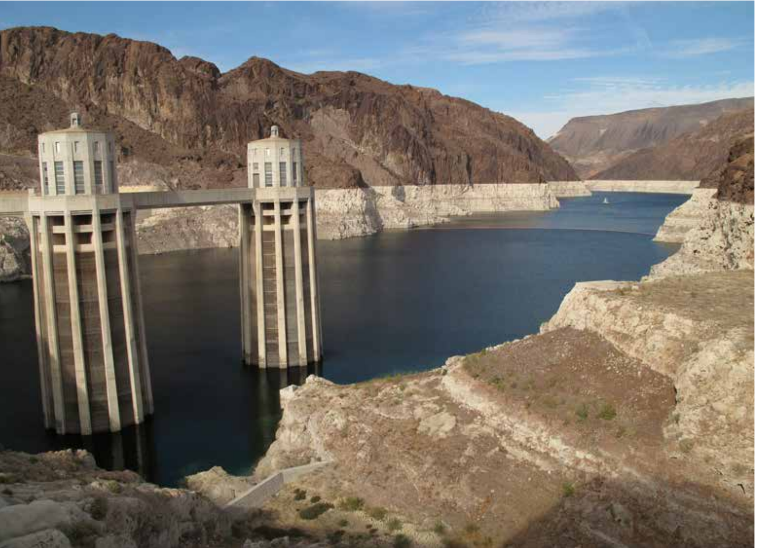
Lake Mead and Hoover Dam water intake towers, as seen from the Arizona side of Hoover Dam, October 2010. WIKIMEDIA COMMONS
